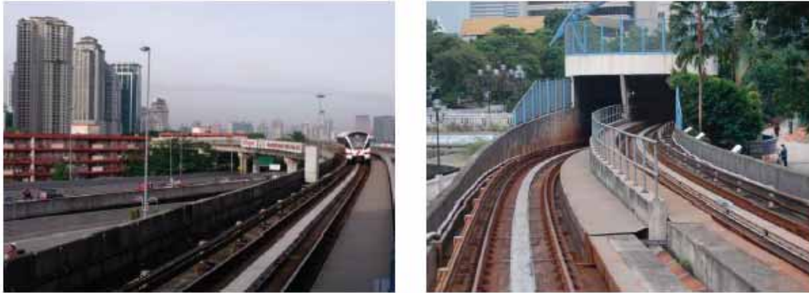
Figure 8: Light rail transit track and tunnel
